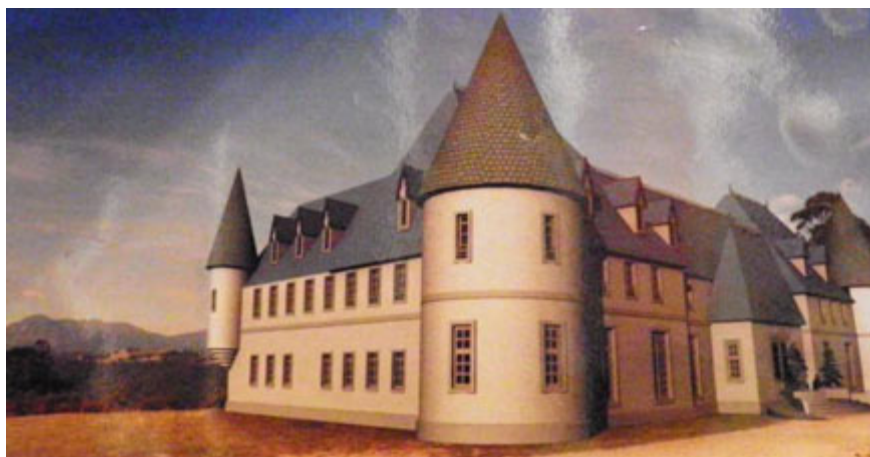
Main Children's Accommodation Building
